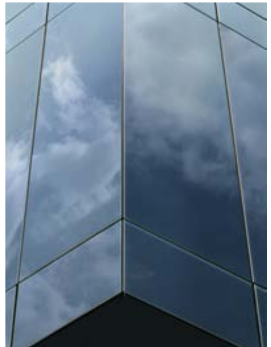
Multiple dwelling, DE-Bad Wildungen; Architect: Gehring & Partner; DE-Bad Wildungen; Photos: Dirk Robbers
