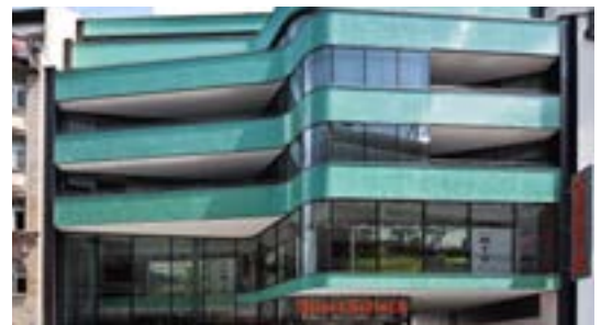
"Royal" residential and commercial building, DE-Frankfurt/Main Architect: schneider + schumacher, DE-Frankfurt/Main; photos: Ben Knabe System: StoVentec M (with glass mosaic)
