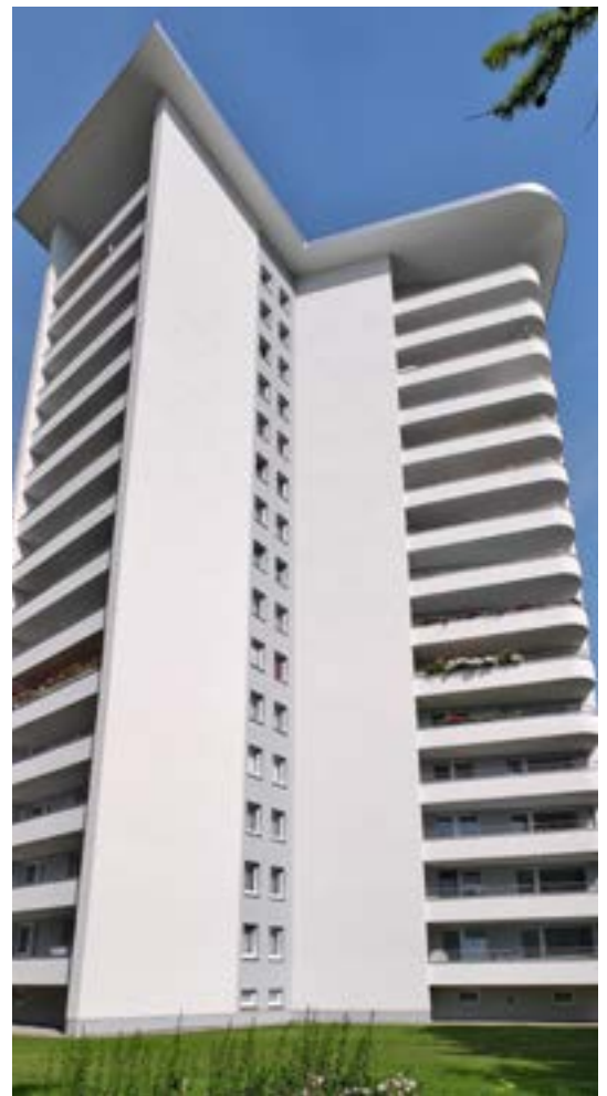
Liebherr high-rise residential building, DE-Biberach
