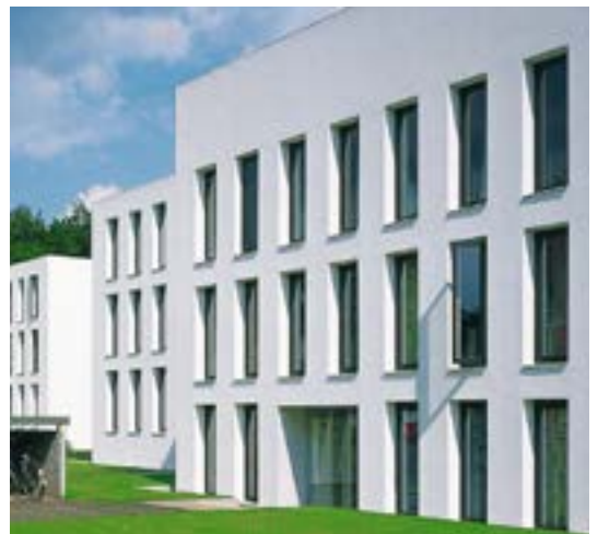
Student houses at University of Twente, NL-Enschede Architect: Claus & Kaan Architekten BNA bv, NL-Amsterdam
