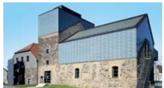
Centrum Bavaria Bohemia cultural information centre, DE-Schönsee; Architects: Brückner & Brückner Architekten, DE-Tirschenreuth; Photos: Guido Erbring System: StoVentec G (with glass)
