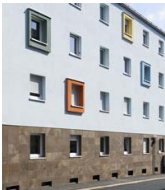
Residential building, DE-Schweinfurt Architect: Architekturbüro Perleth, DE-Dittelbrunn
